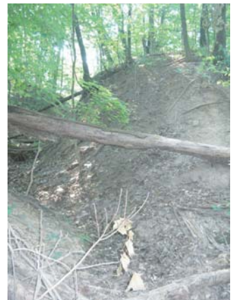
Steep ravines form with concentrated runoff and a lack of appropriate vegetation to hold soil in place.
