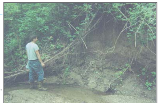
Streambank erosion in Tenmile Creek is a major source of sediment for Peoria Lakes.
