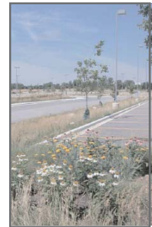
Engineered swales such as those suggested in the Unified Stormwater Ordinance filter and infiltrate stormwater (above).
