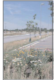
Engineered swales such as those suggested in the Unified Stormwater Ordinance filter and infiltrate stormwater (above).
