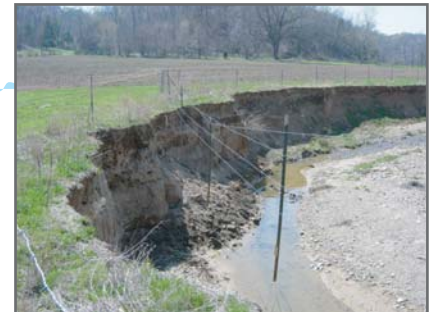
This photo demonstrates the magnitude of soil loss from streambank erosion.
