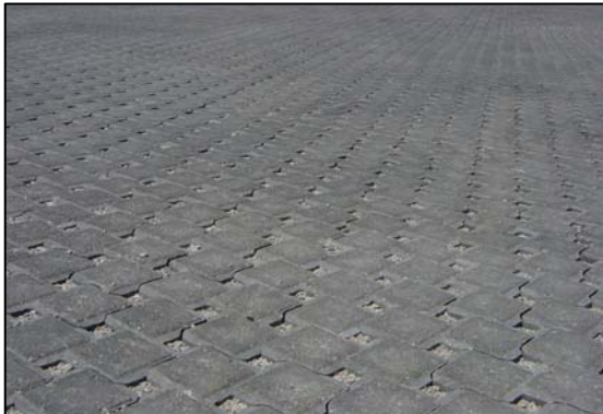
Fig. 7 Porous pavement in a community college parking lot.
